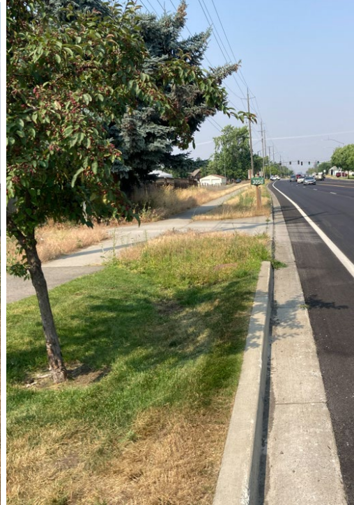
Curb and sidewalk at 3050 Prairie Ave.
