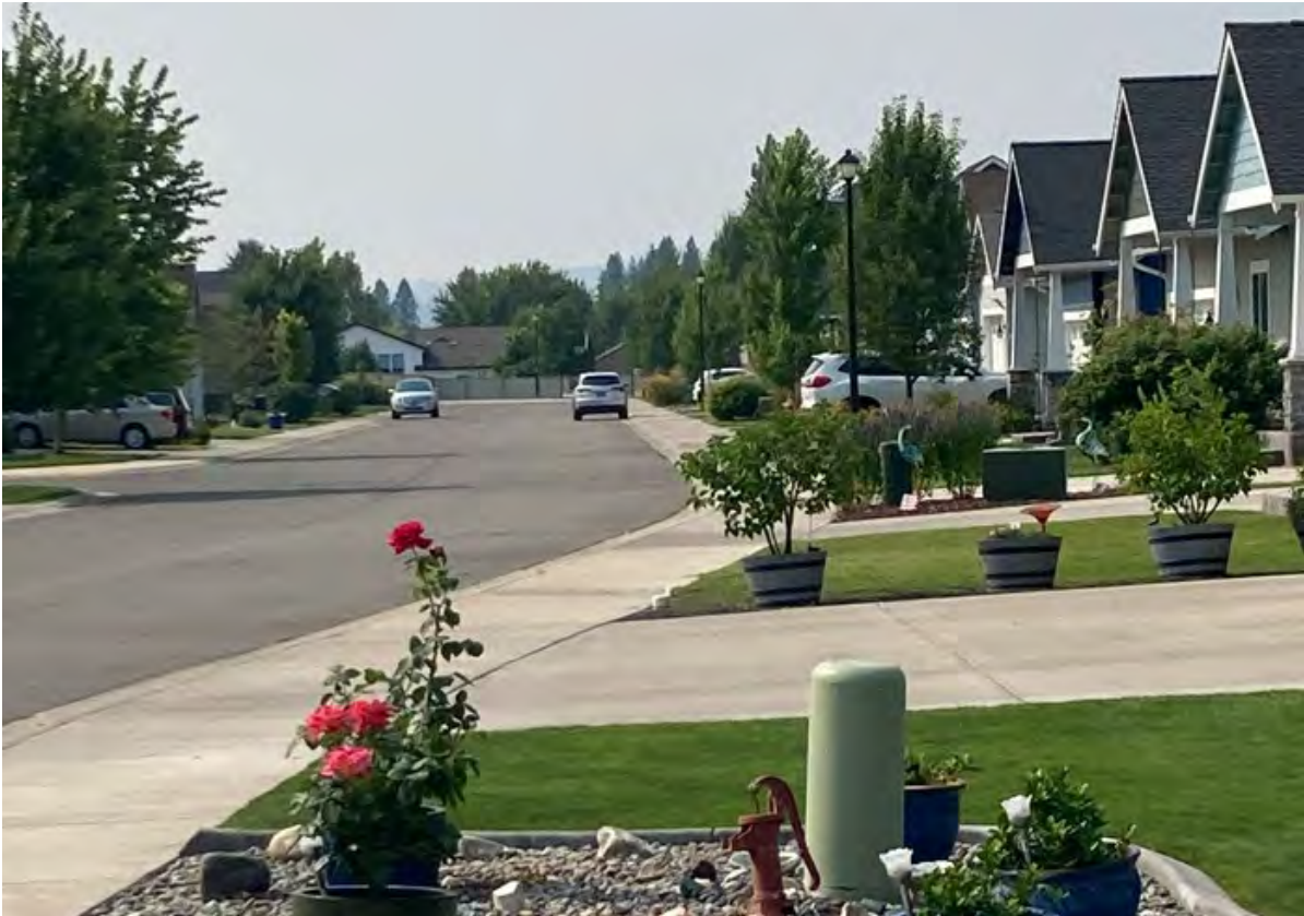
Typical roadway, curbs, sidewalk
