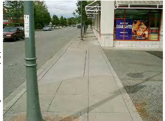
Sidewalk pavement is visibly continuous
