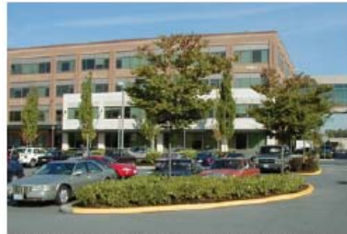
parking lot located behind commercial building
