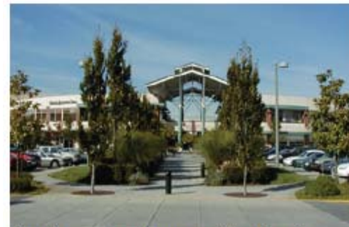
visually prominent entrance with pedestrian connection
