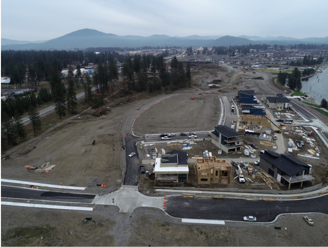
SITE PHOTO 7 - Drone Photo Looking at Areas 1, 2, 8 and 10:
