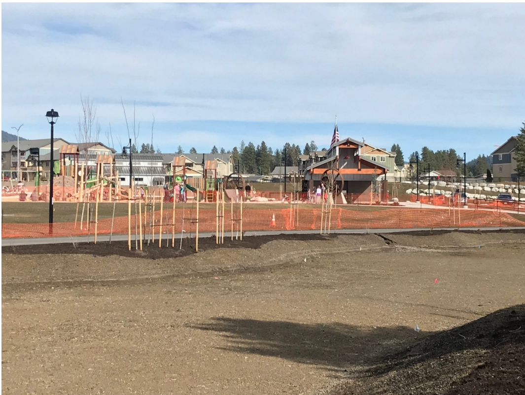
SITE PHOTO 2 – Atlas Waterfront Park and Swale:
