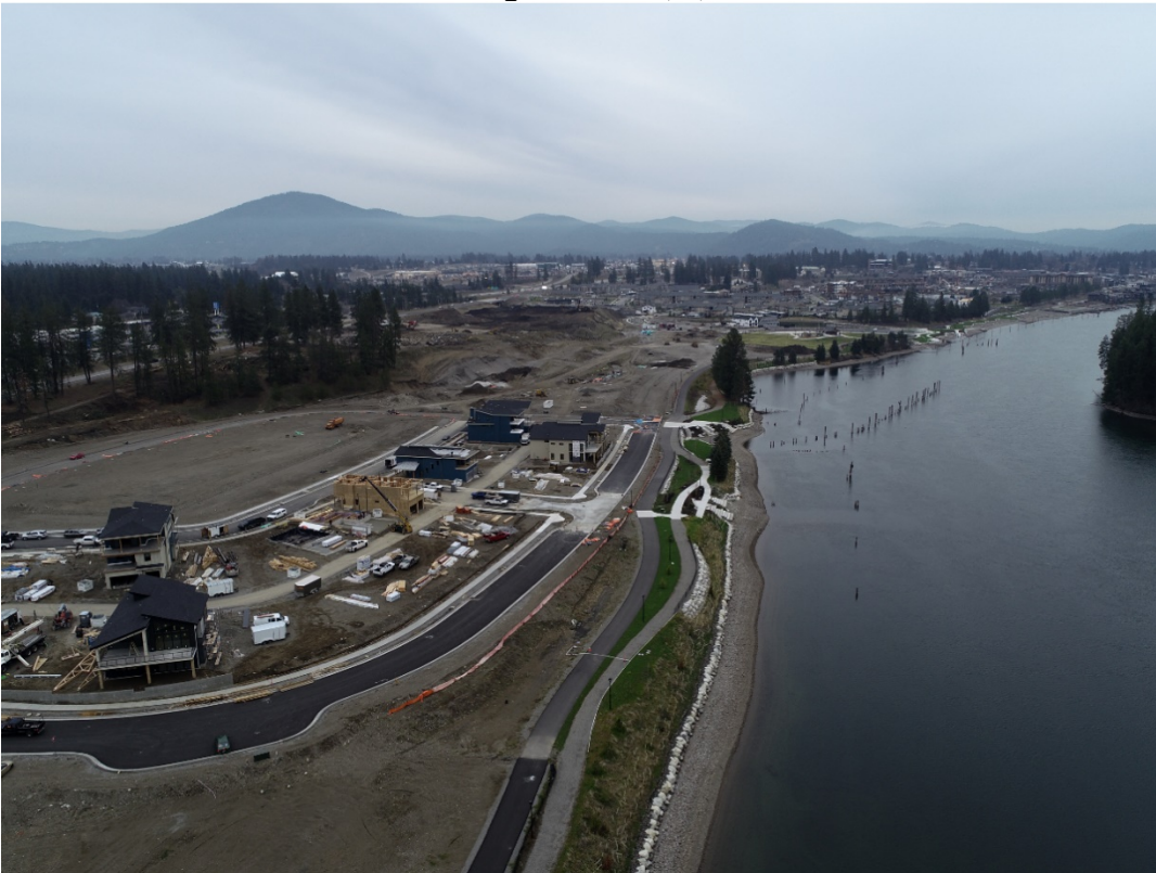
SITE PHOTO 6 - Drone Photo Looking at Areas 1, 2, 8 and 12:
