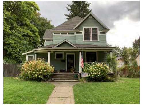
Figure 33. 522 E Indiana Avenue
