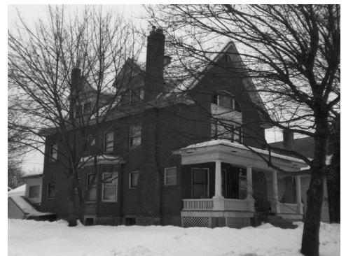
Figure 39. 315 Wallace Avenue Colonial Revival example. Courtesy National Park Service.
