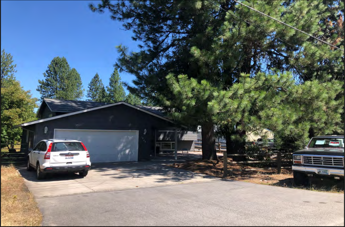
View of the subject property looking south at the existing single family dwelling unit.
