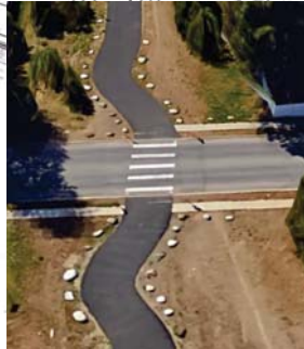
Option 2 would be similar to the Prairie Trail Crossing at Player Drive
