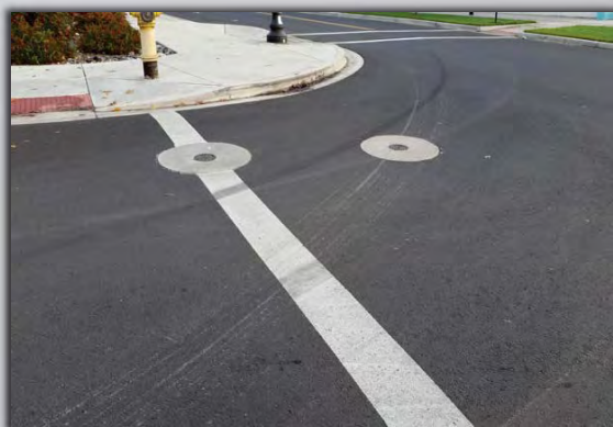
City of Lewiston Water Valves (Single)
