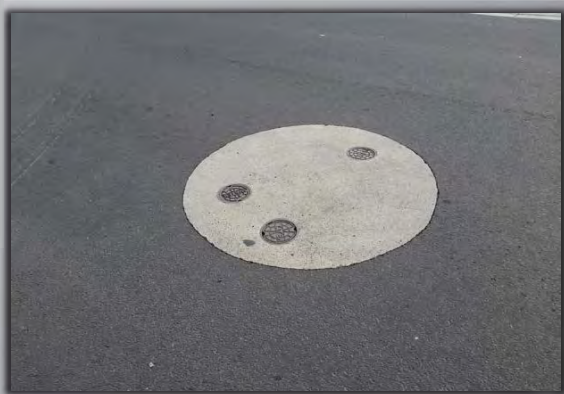
City of Lewiston Water Valves (Cluster)
