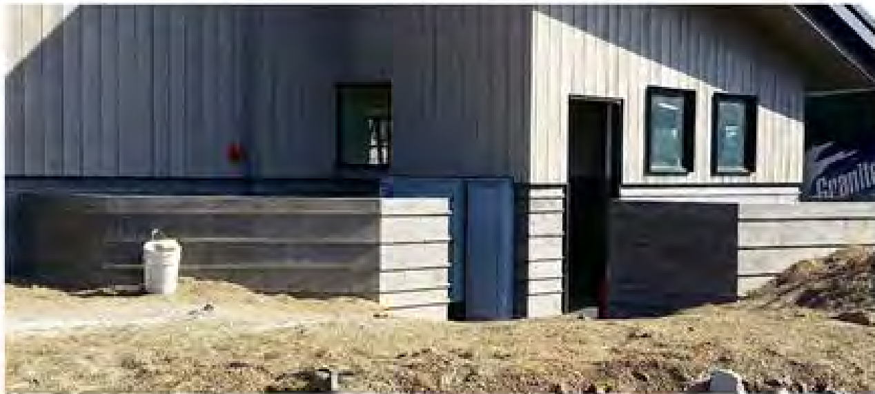
PROPOSED EXTERIOR FINISH CONCRETE WALL SAMPLE
