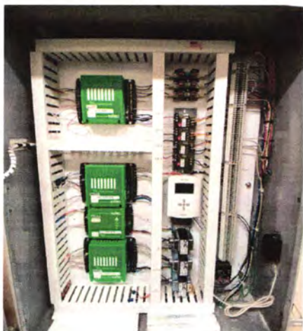
Existing temperature control panel
