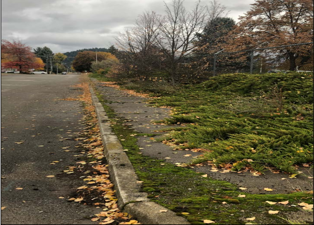
VIEW ALONG THE GOVERNMENT WAY ACCESS POINT LOOKING EAST AT THE EXISTING SIDEWALK
