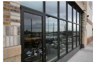
EXT. WINDOW SYSTEM: METAL STOREFRONT SYSTEM COLOR: 'BLACK' OR APPR.
