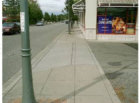
Sidewalk pavement is visibly continuous
