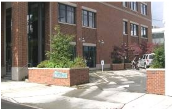
Parking Located To The Side
