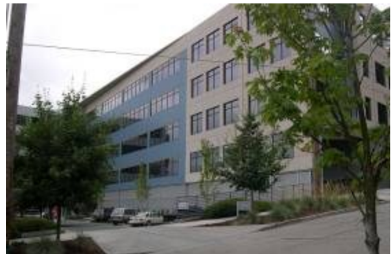
Parking Located Behind
