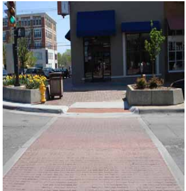
Another example of using color and texture to create a clear path for pedestrians. This example uses planters to protect pedestrians waiting to cross the road.
