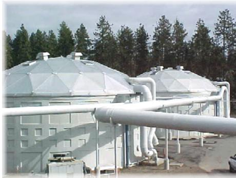
1995 - Plastic Media Trickling Filters and Foul Air Ducting. Foul air is pretreated in the trickling filters.
