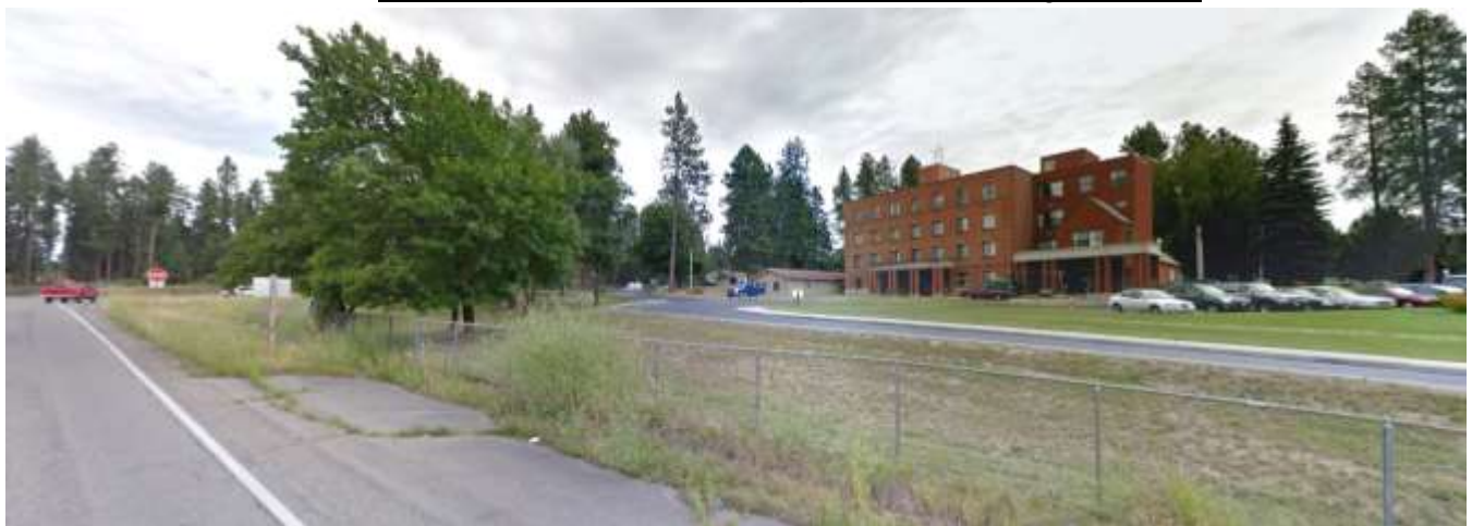
Northwest Boulevard exit ramp to US 95 looking northeast
