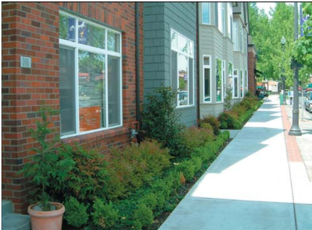
Examples of Acceptable Siding Including Brick, Cedar Shake and Traditional Lap Siding
